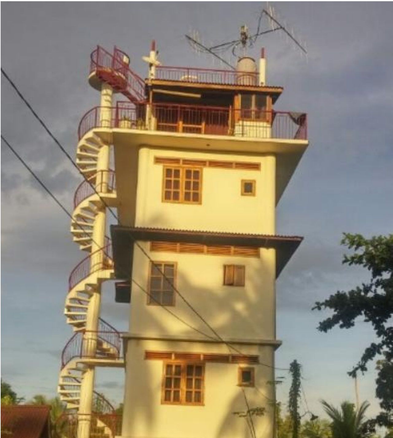
Antennas and shack were on top of a 16 m tower (Photos DX7EME)
